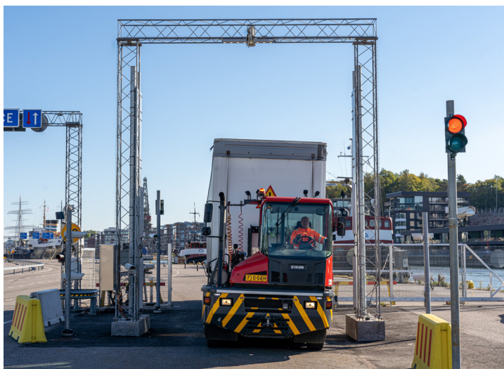
Pre-gate area with Visy IRIS OCR Portal and traffic guidance equipment
