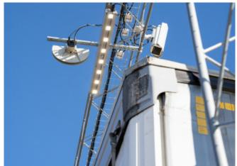
Visy OCR Portal captures images and identification data from all sides of containers, making the flow of traffic more transparent and automated
