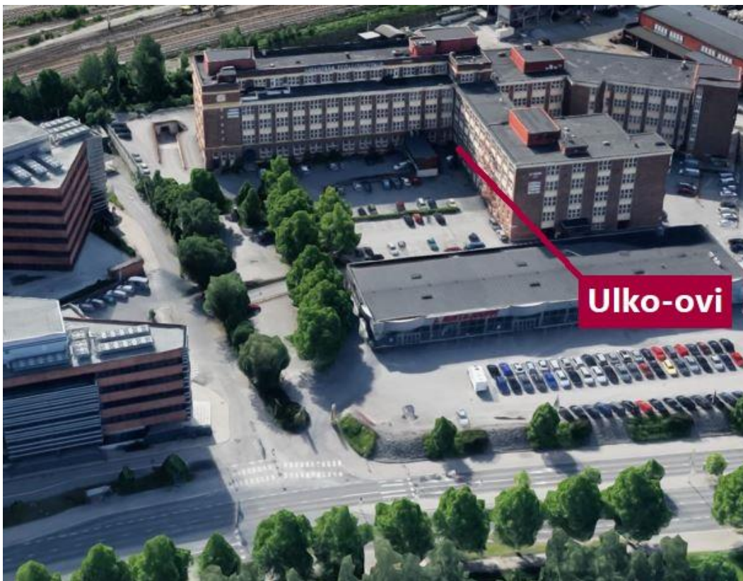
Door to the D-stair (Package delivery / pick-up)
